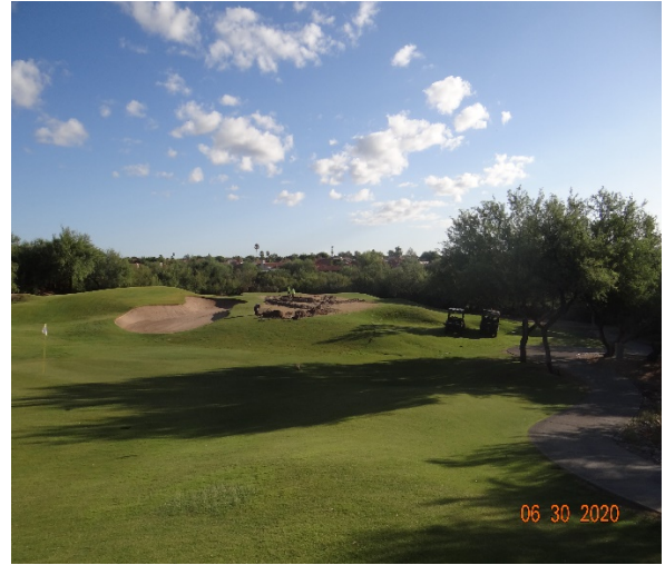
#17 – Exposing Flat Drains
