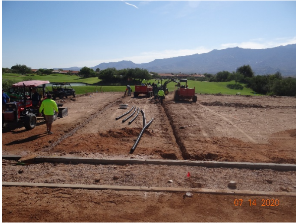
Driving Range Drainage Being Installed
